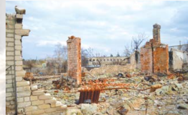
Remains of a residential building on Ostrovskogo Street after the airstrike
