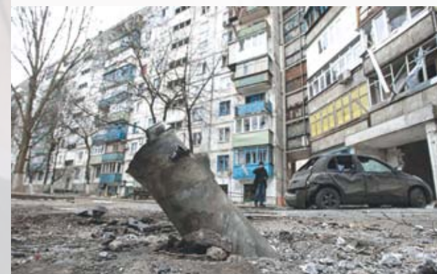
Skhidniy block in Mariupol after the shelling
