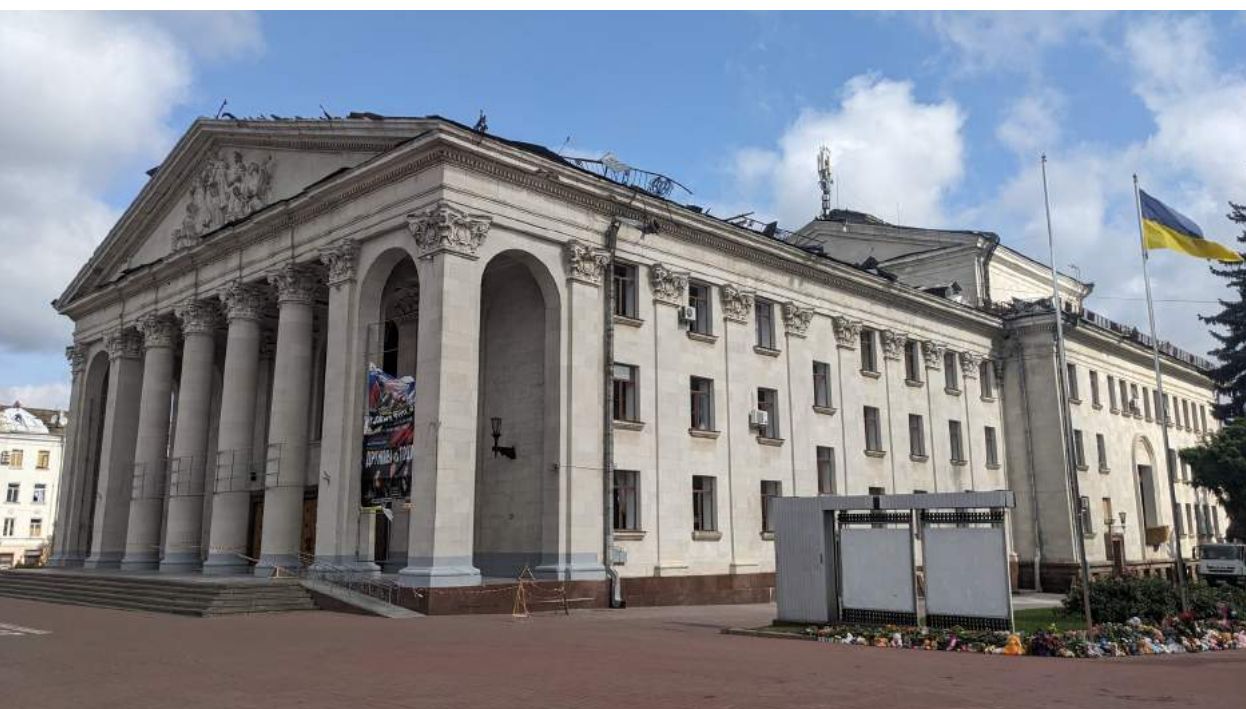
The theater building in Chernihiv damaged by a missile strike, 22.08.2023. Photo source: EUCCI
