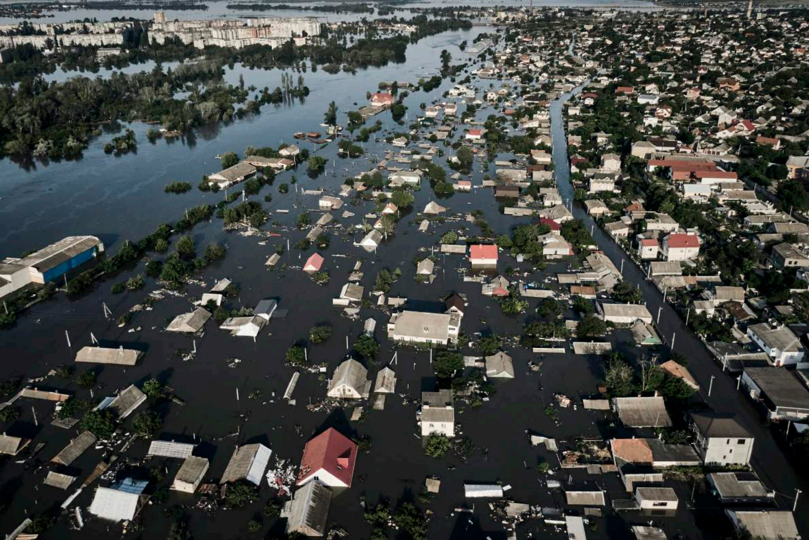
Streets of Kherson after the destruction of the Kakhovka Dam. Photo source: alamy.com
