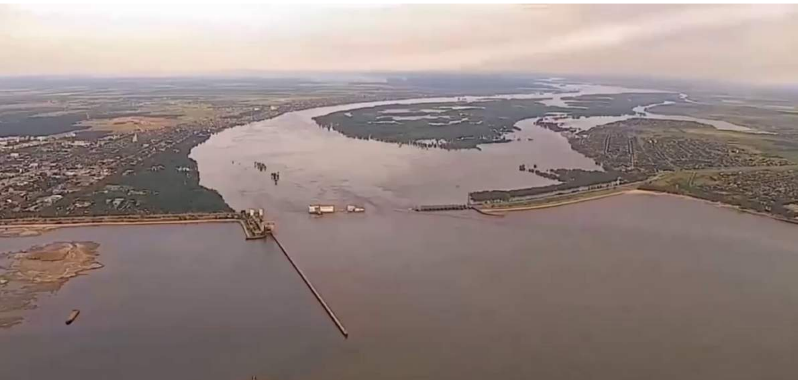
The Kakhovka Hydroelectric Station after its destruction. Video screenshot. Source: Ukrainian news / State Border Control Service of Ukraine
