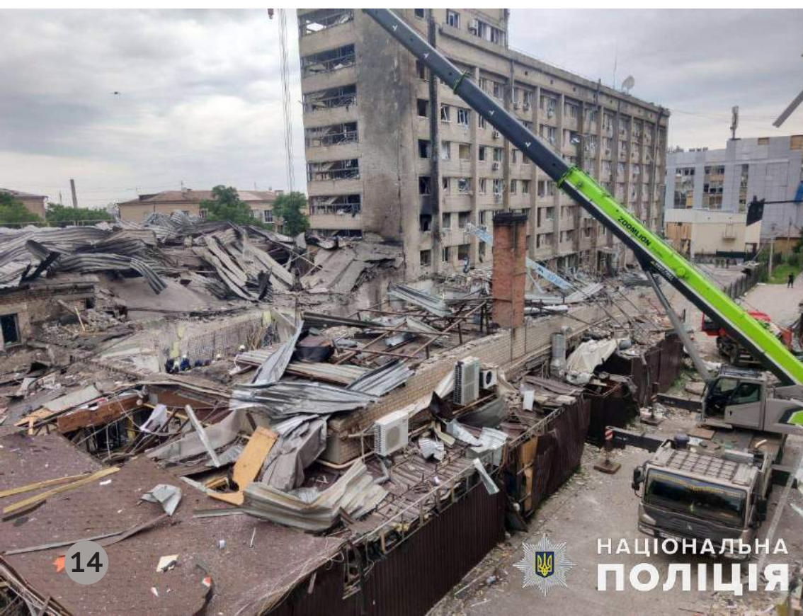
The building of the café-pizzeria in Kramatorsk, 27.06.2023. In the background the building of the hotel "Kramatorsk" can be seen. Photo source: National Police of Ukraine
