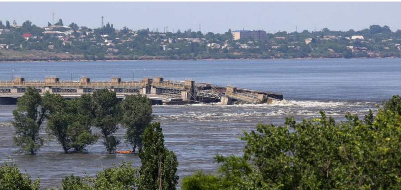
Flooding in the city of Kherson as a result of the destruction of the hydroelectric station. Photo by REUTERS / Oleksandr Klymenko. Photo source: NV.UA
