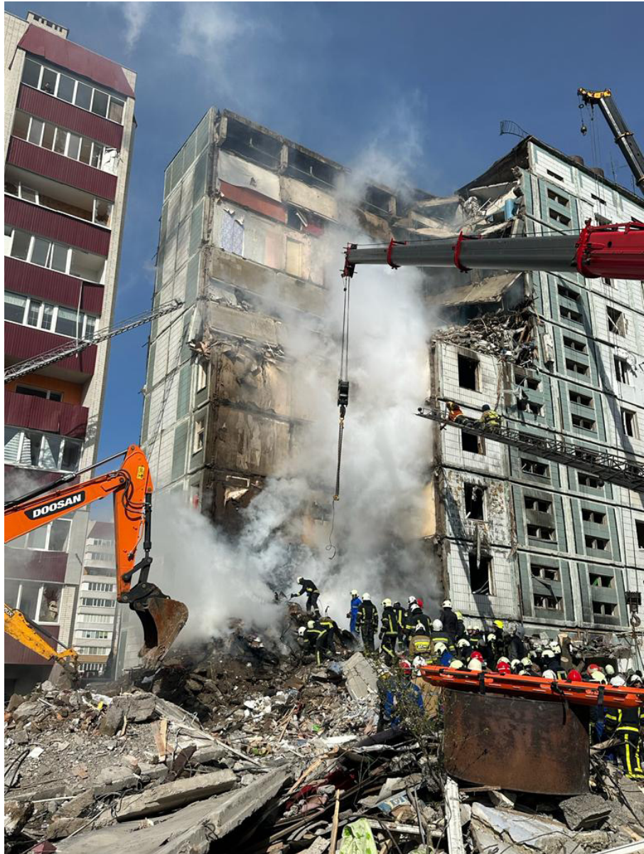
Rescuers sort through the rubble of a nine-story apartment building in the city of Uman after it was hit by a Russian missile. Photo source: State Emergency Service of Ukraine.
