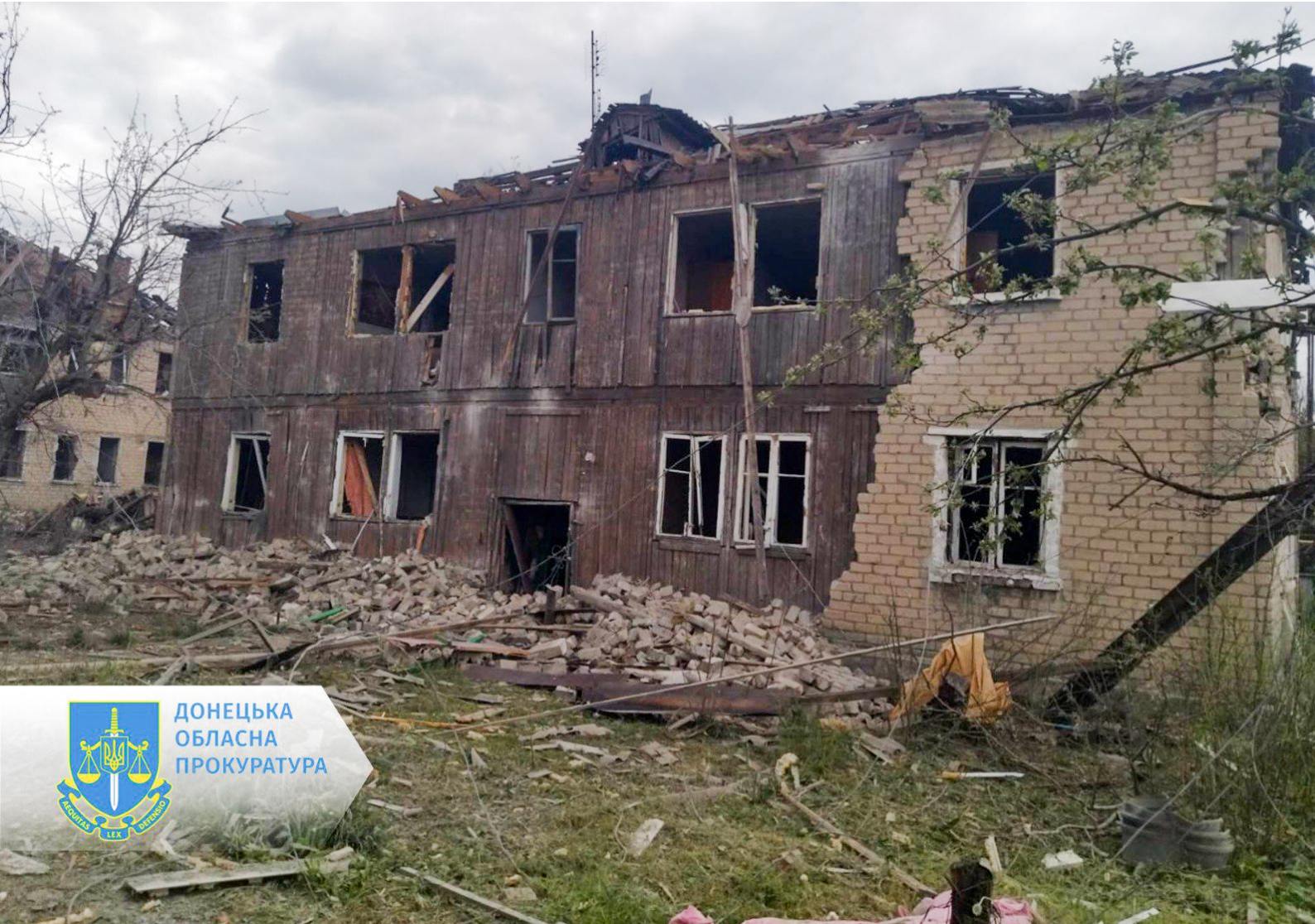
Residential buildings in Toretsk after the shelling, 11.05.2023. Photo source: Office of the Prosecutor General and Donetsk Regional Prosecutor's Office.
