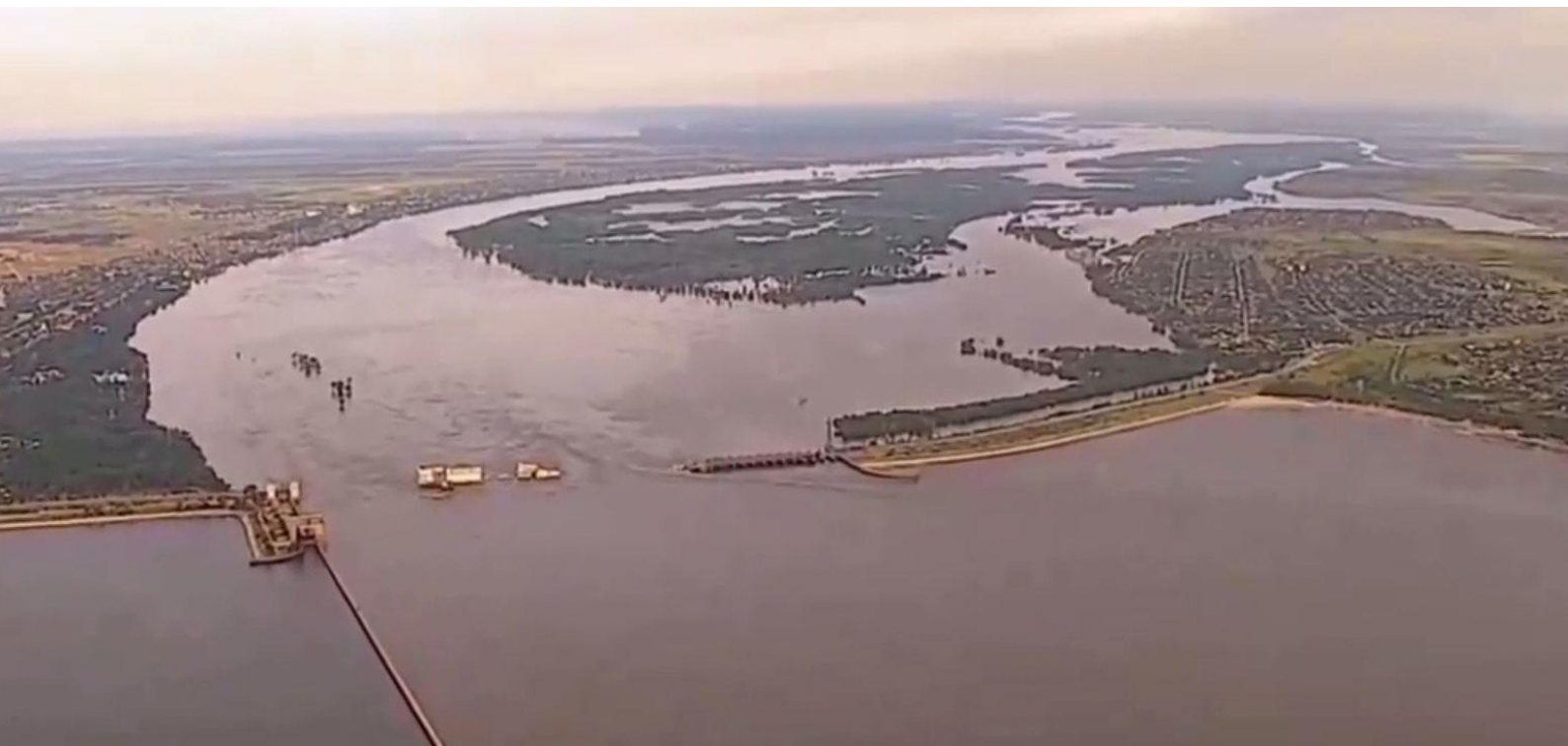
Kakhovka dam after destruction. Video screenshot. Source: Ukrainian news/State Emergency Service
